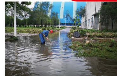
Qinbei Power Plant Conducted Drainage Work in Low-lying Area
