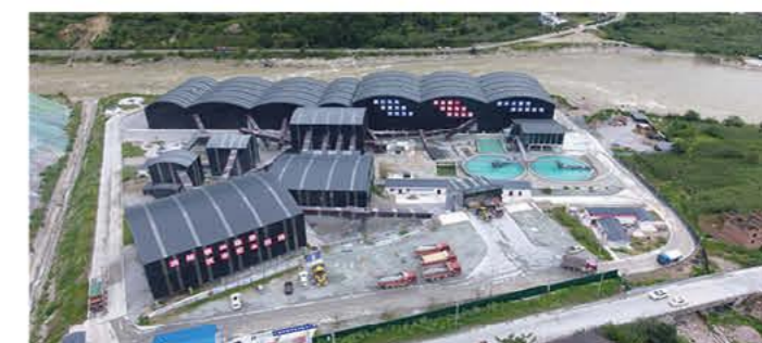
Aggregate Processing Area of Yingliangbao Hydropower Station
