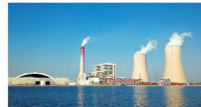
Huaneng Sahiwal Coal-fired Power Plant
