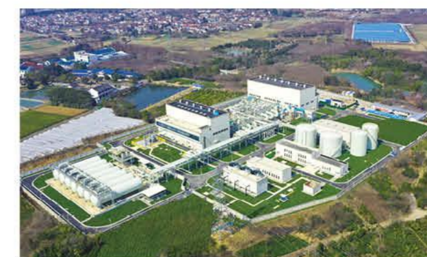
Jintan Salt Cavern Compressed Air Energy Storage Project
