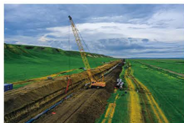
The World's Longest Yimin-to-Hailar Underground Heating Pipeline in the Alpine Region
