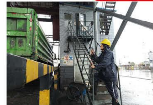
Luoyang Thermal Power Plant Strictly Controlled Moisture Content in Coal Yard
