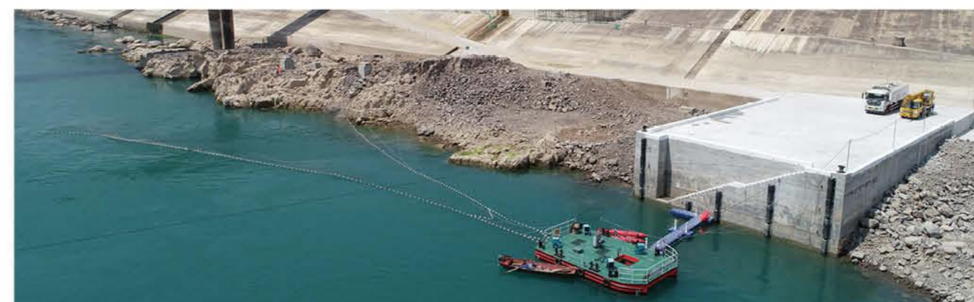
First Large-scale Hydropower Station Fish Collection and Transportation System in the Stem Stream of the Yangtze River
